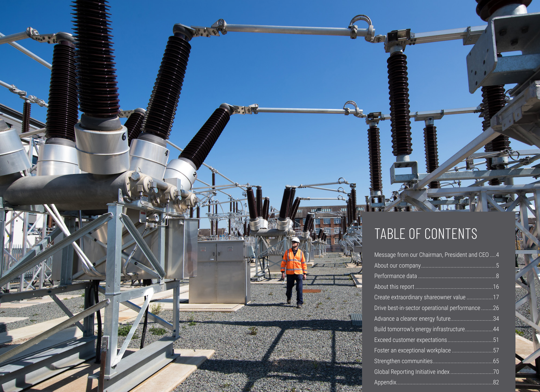
A WPD employee inspects a substation.
