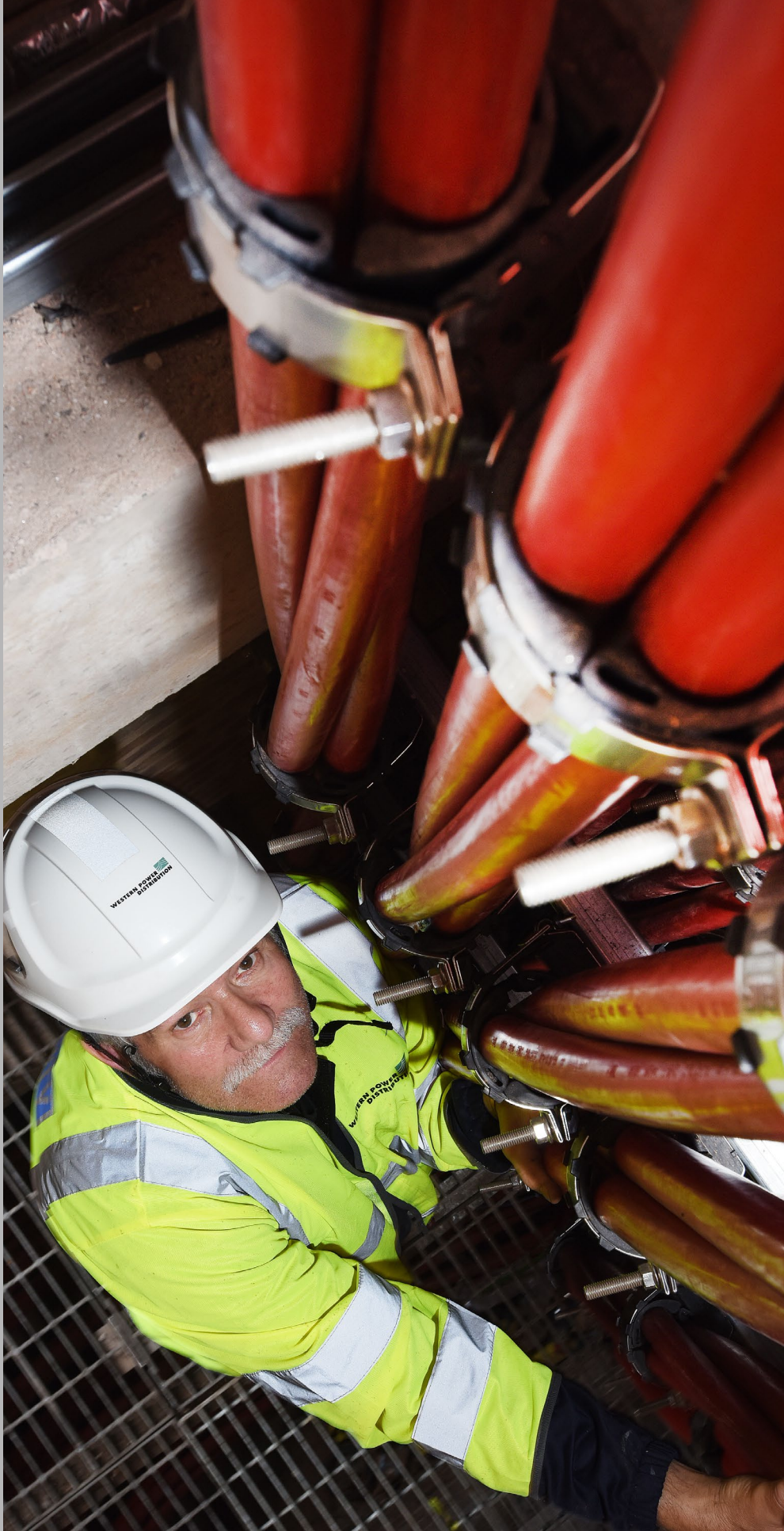
A WPD EMPLOYEE INSPECTS NEWLY-INSTALLED HIGH VOLTAGE CABLES IN AN EXISTING RISER SHAFT AT THE WINSON GREEN 132/11KV SUBSTATION.
