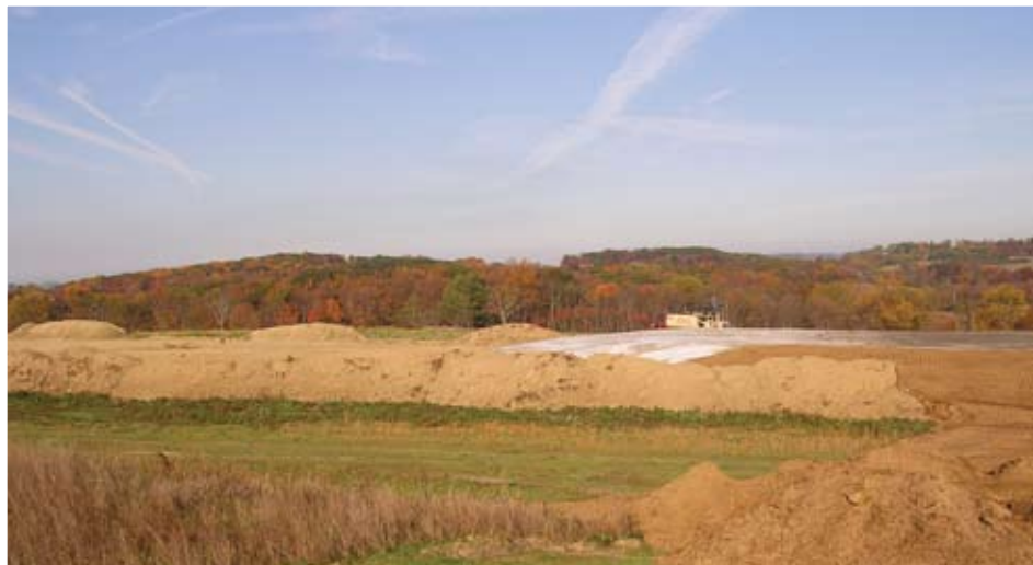
Environmentally safe Stabil-Fill helps shape the recreation complex in Madison Township.
