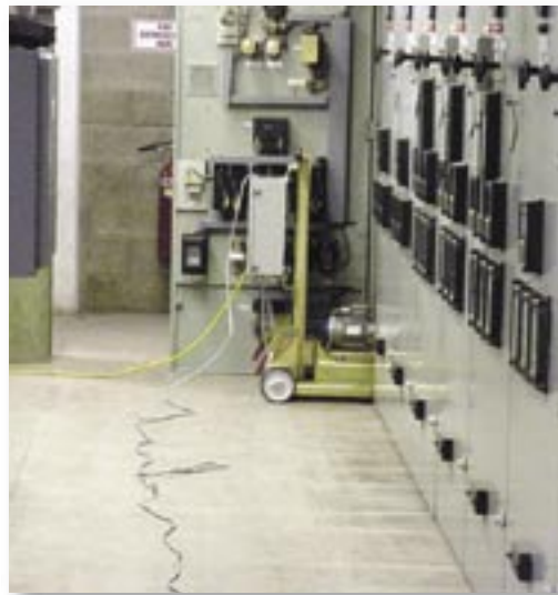
A remote racking machine safely removes and installs breakers.
