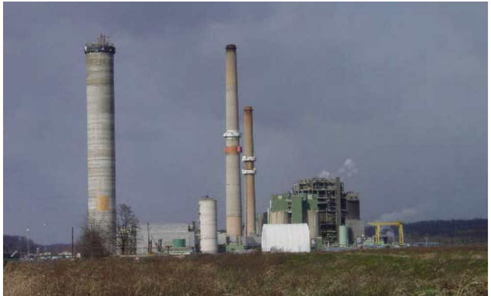
A 580-foot concrete chimney stack (left) is now complete at the power plant.
