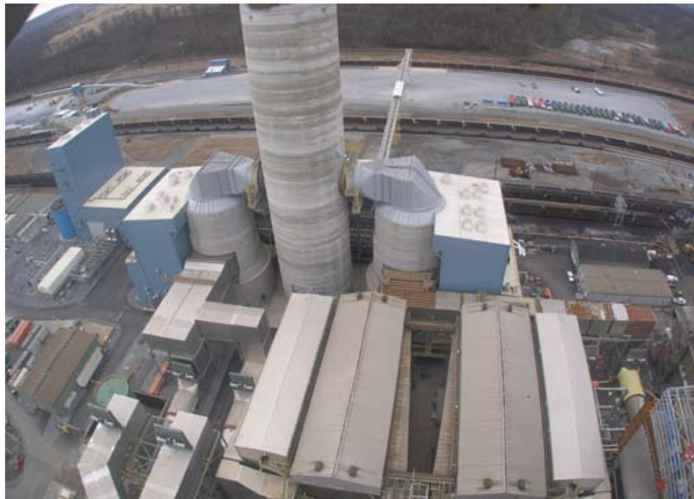
The first of two scrubbers, designed to improve air quality, will be in operation this spring.
