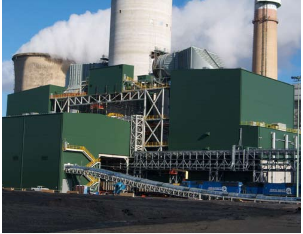
An overall view of the scrubbers on Units 1 and 2.
