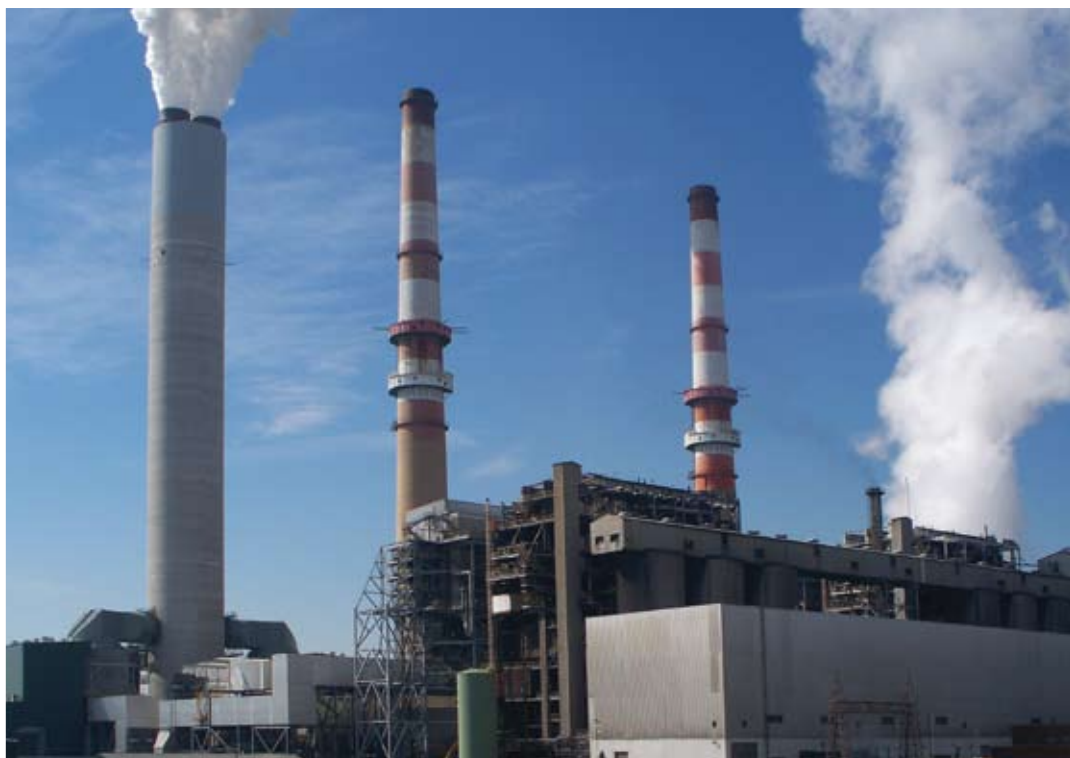
White, cloudlike plume contains mostly water vapor and signals that the scrubber is doing its job for the environment.
