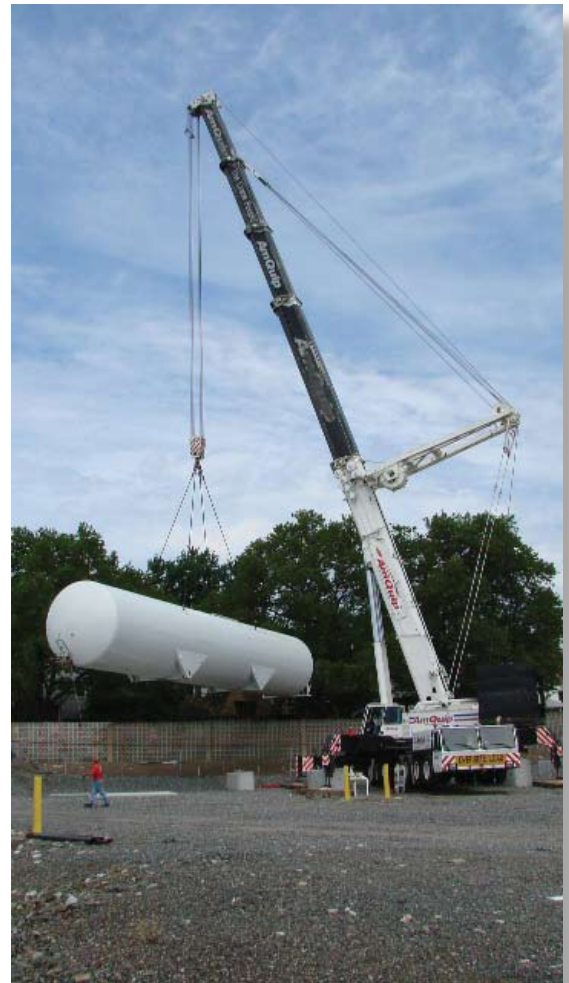
A 500-ton crane was needed to lift the nitrogen storage tanks.
