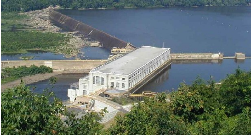
Photo 4-1. Holtwood powerhouse and dam (taken from east side of river).
