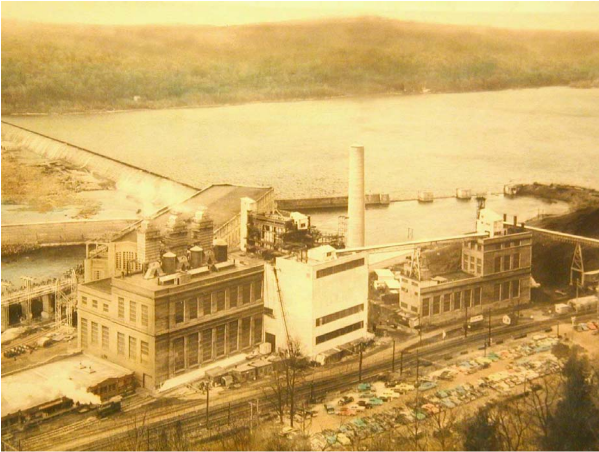
Photo 5-1. Steam station that occupied area of current proposed development.
