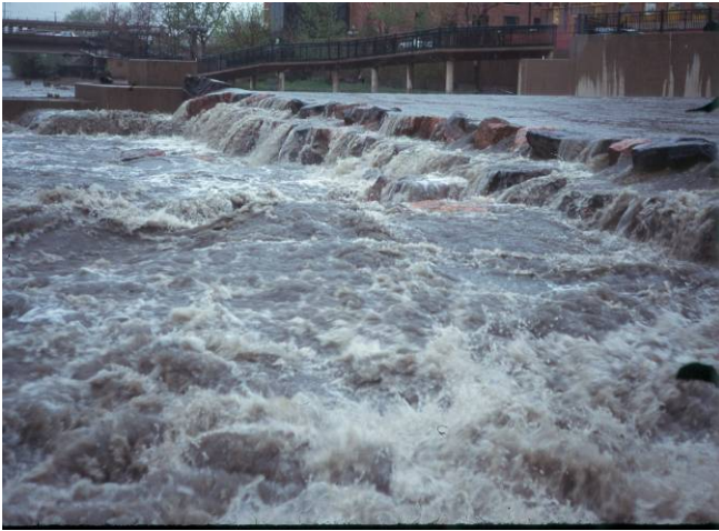
Figure 10 One of Four Dams Specifically Designed to Eliminate “Keeper” Hydraulics. This Dam has Operated for Eleven Years in Downtown Denver without Mishap or Maintenance.
