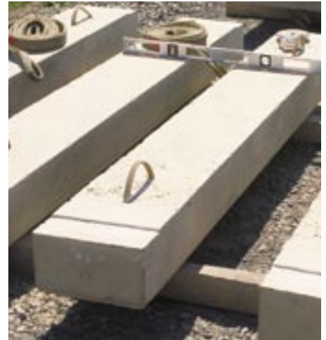
The wooden stop logs have been replaced by these steel-reinforced concrete logs.
