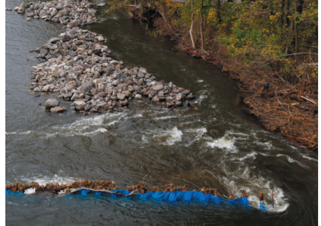
The portable dam was visible again as the river level dropped.
