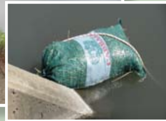
Bruce Lamotte, a chemical technician for the Montour plant, holds an onion bag filled with straw used in a stormwater retention basin. The basin filters rainwater running off parking lots and field areas before it is discharged into the Chillisquaque Creek.
